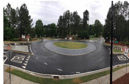
Road Construction $26M
