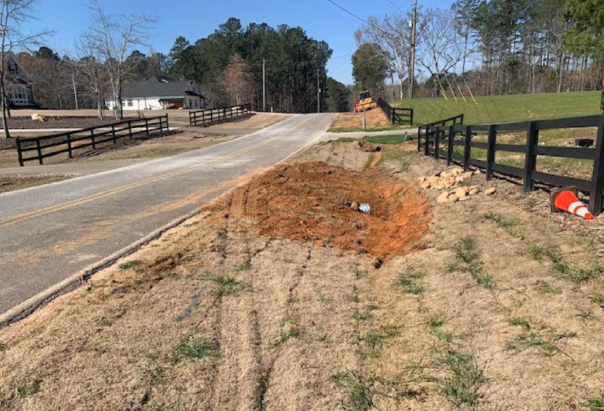
MT CARMEL CHURCH—PUBLIC WORKS
