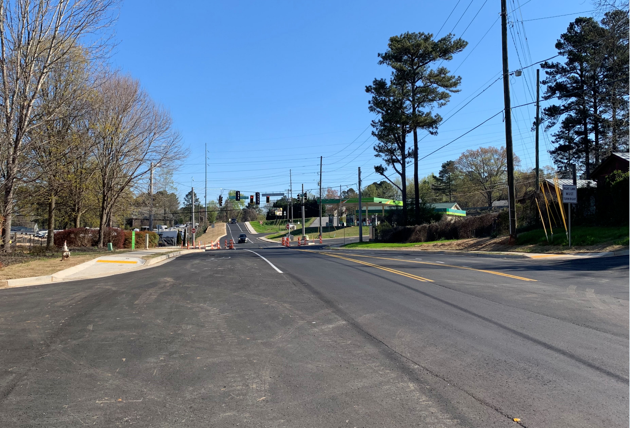
BELLS FERRY ROAD AT KELLOGG CREEK ROAD AT VICTORY DRIVE INTERSECTION IMPROVEMENT
